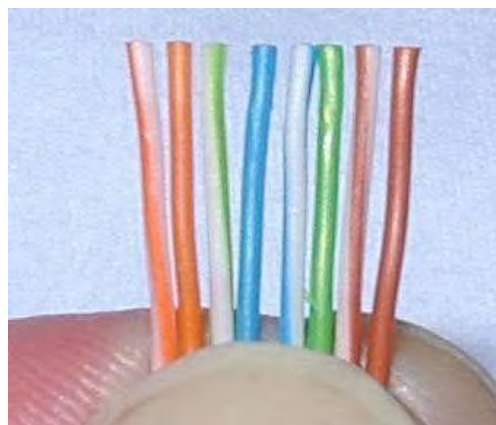
Fig 1.9 Straighten wires with fingers
